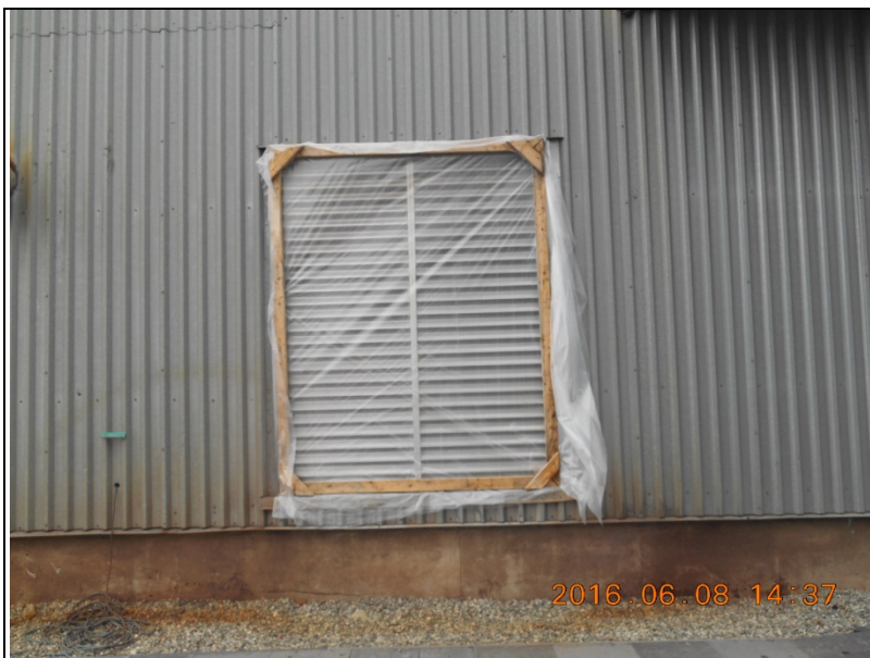
Fig. 7: Stator Louver protected with plastic to reduce moisture in the windings
