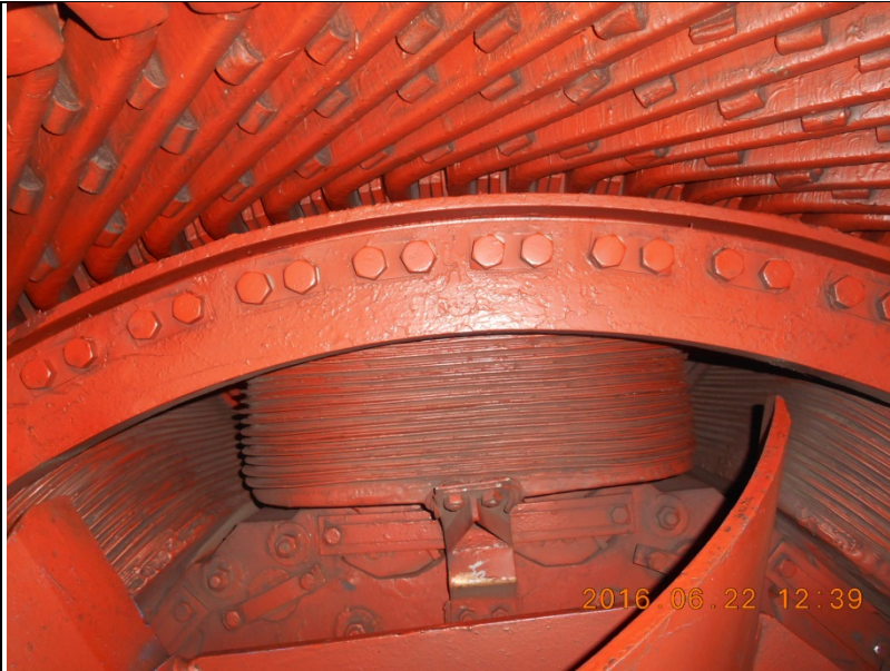
Fig. 11: NCRE Damper winding -.
