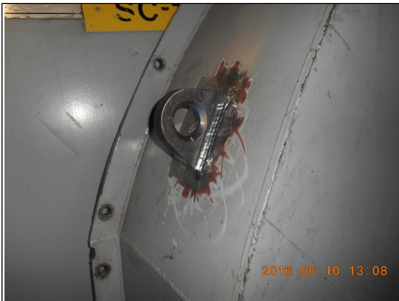
Fig. 27: New lifting lug installed
