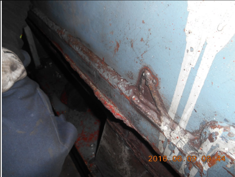
Fig. 3: Collector End Bearing Pedestal - Oil film and metal shavings accumulated on isolation pad
