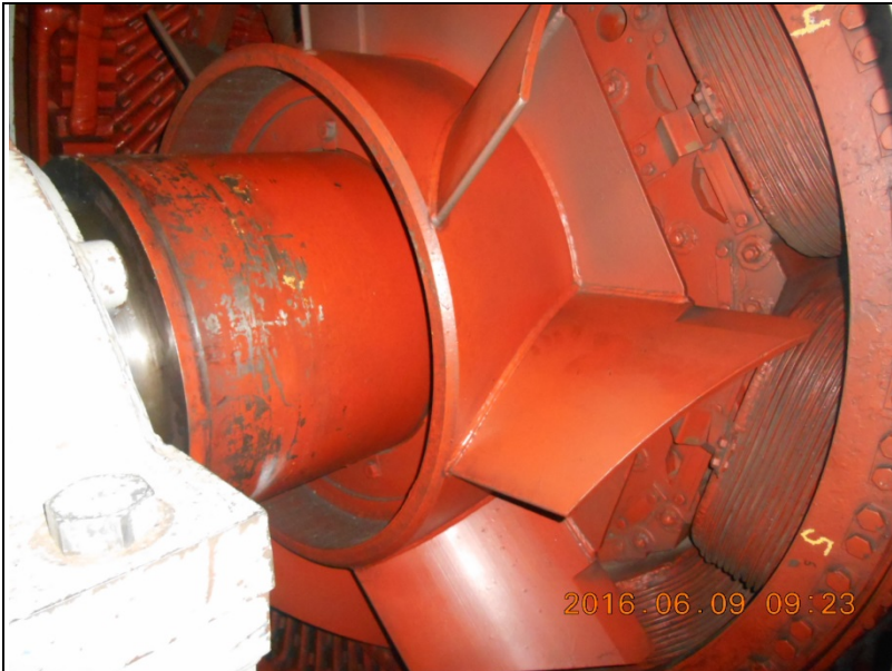
Fig. 8: Collector End - View of rotor poles and fan
