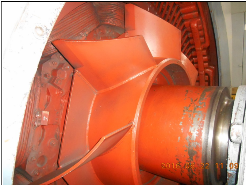
Fig. 6: Collector End - View of rotor poles and fan
