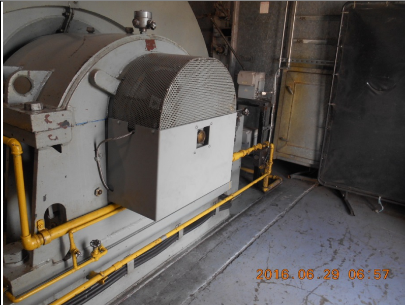
Fig. 31: SC2 NCRE Thrust End - New guard installed
