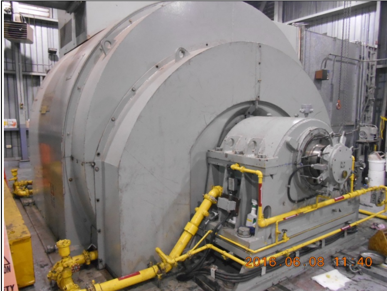
Fig. 4: The oil film appears to be a result of small leaks in the external oil piping. There are a number of oil absorbing pads placed on the outside of the bearing pedestal and around the unit.
