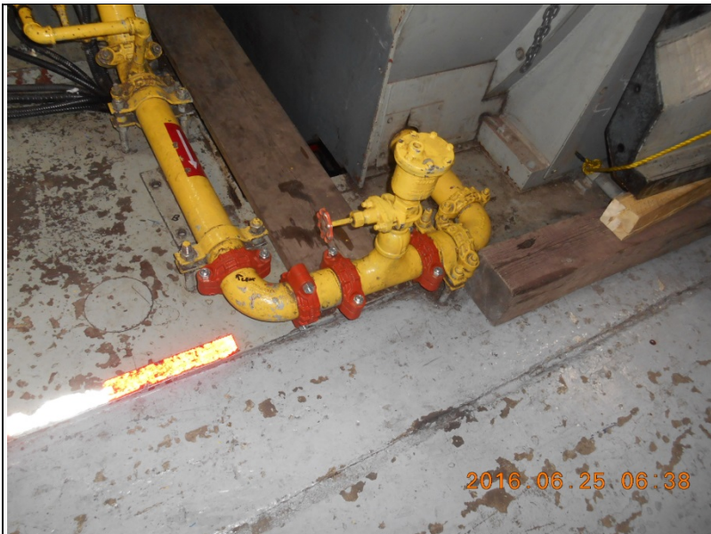
Fig. 3: First section of Victaulic Couplings replaced (orange) to correct oil leaks
