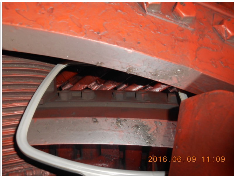
Fig. 10: Inspecting the back side of the damper winding with a mirror
